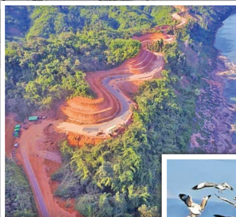
Myitkyina-Putao-Sumprabum Road being upgraded in Kachin State.
