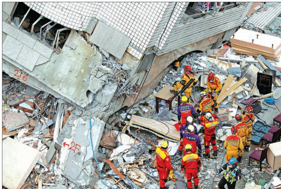
Rescue personnel work at a collapsed building after an earthquake hit Hualien, Taiwan, on 9 February 2018. PHOTO: REUTERS
